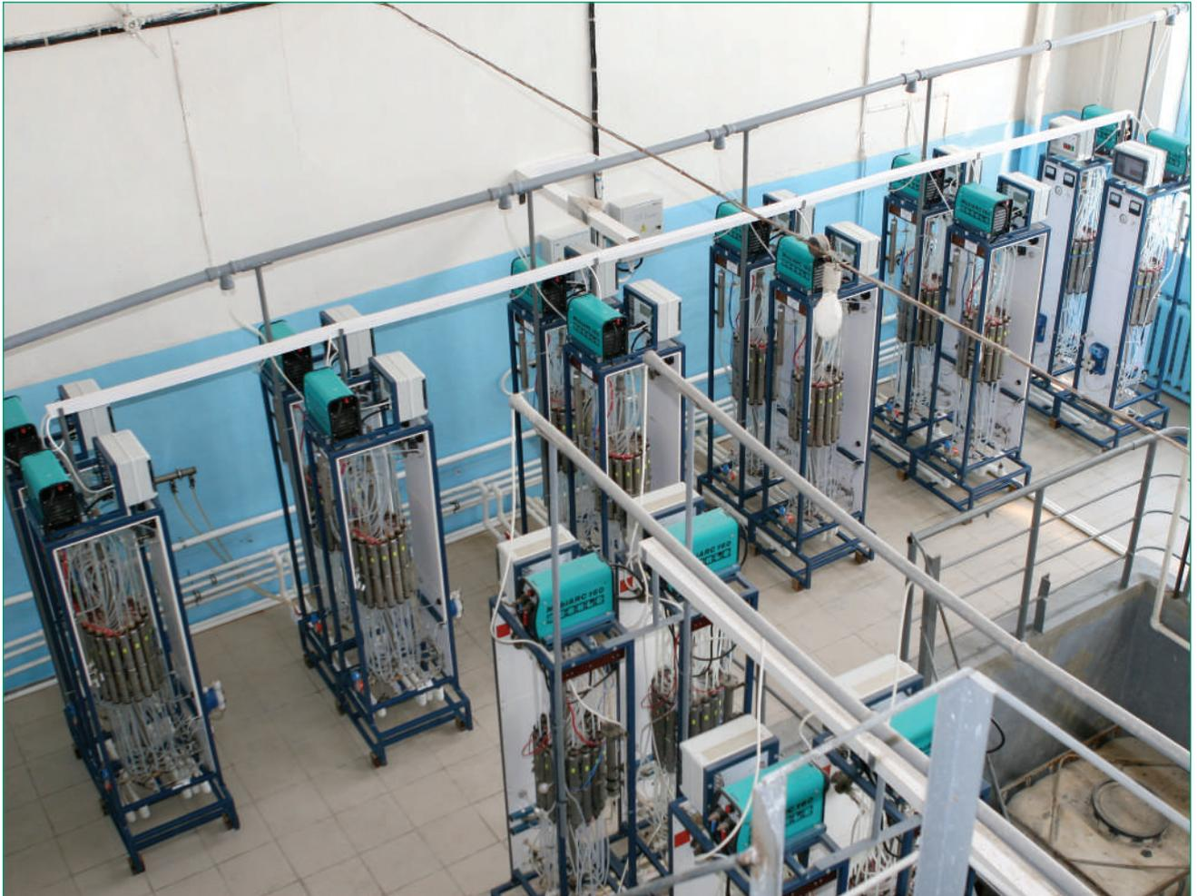
*Fig. 5.6.5. AQUACHLOR-500 devices at the Balakovo water treatment system. In total, the system uses 76 A-500 devices, including standby ones. The daily productivity of the system in molecular chlorine equivalent is more than 900 kg.*
